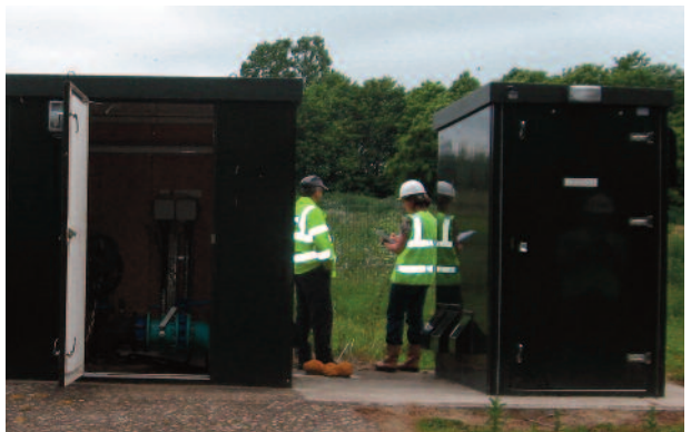
Huts are the only visible structure at permanent ASR sites
